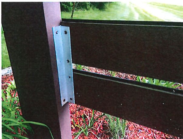
Back side of signs 3/4" particle board structure with aluminum L bracket Face of sign mounted to particle board
